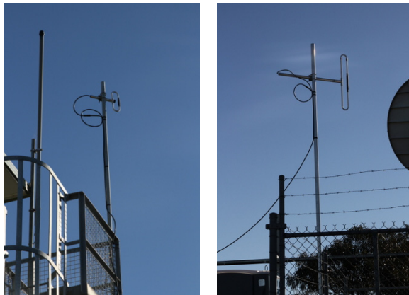
Below: UHF repeater antenna and VHF translator antenna at Mt Ida
